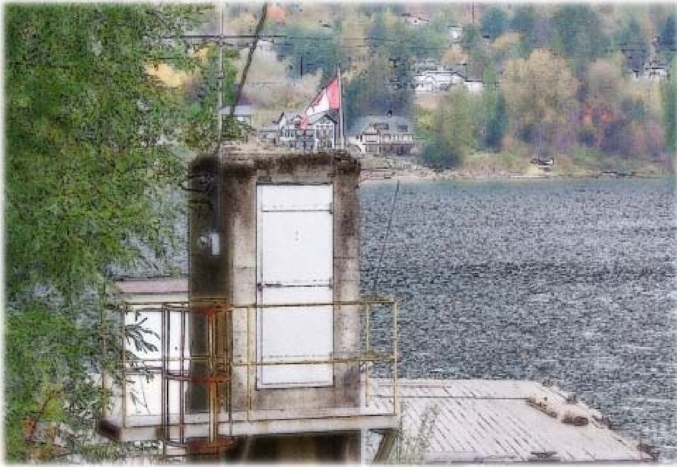
Nelson Water Level Gauge House
