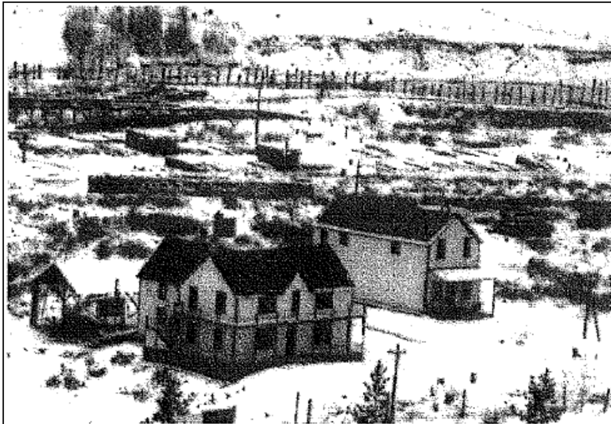
Bunkhouse in fore ground with the store on the right. The river pylons can be seen in the background. Source: Greg Nesteroff, detail.
